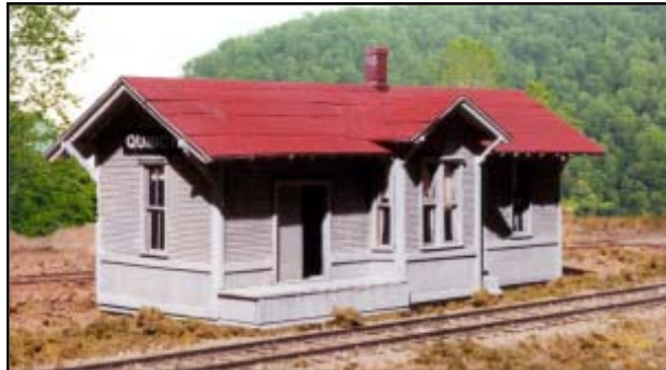
DT&I Standard Station, Waiting Room Right
